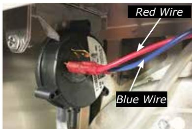
13. Bundle the wires together with the supplied grommet and pop the grommet with wires into the bracket on the roof of the power vent box.
