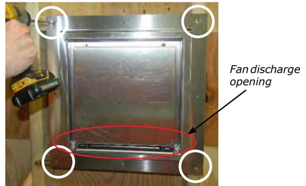
9. Seal the edges of the Power Vent unit to the framing (there are two seams).
