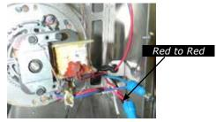
17. Connect remaining wires from the power vent motor to the BX cable- black to black and black to white. Cap paired wires with supplied marrette.
