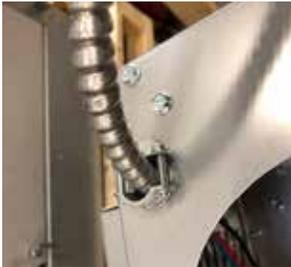
3. Tie the supplied zip tie loosely as shown below and pop it into the wall of the power vent box. Bring blue/red wires from the BX through the zip tie.
