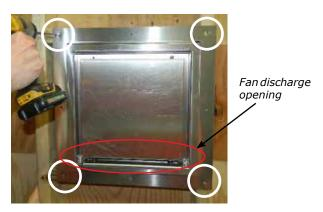
9. Seal the edges of the Power Vent unit to the framing (there are two seams).
