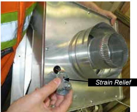
4. Strip the sheath from the BX cable to expose approximately 8" of exposed wires.
