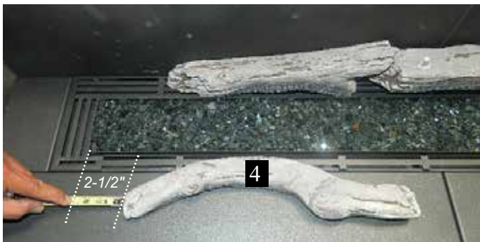
Log 4 to edge of burner
