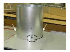
5. Connect the flex pipe to the adaptor with 3 screws.
