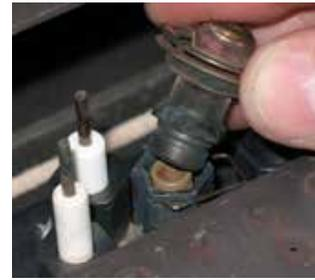
16. Unscrew the pilot orifice with the Allen key; then replace with the LPG pilot orifice and the pilot cap, provided in the kit.
