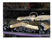
17. Install Log 10—line up the pin locator on Log 10 with the pin on Log 1 and rest the other end of Log 10 on the rest on Log 5 as shown below.
