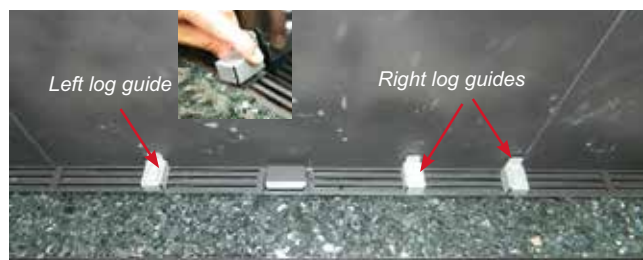
Log guides installed
