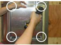
Loosen 4 screws in locations shown below, lift rain guard off screws (key hole slots).
