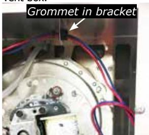
14. Install the second grommet onto the wires and secure grommet and wires into a bracket located on the side of the power vent box.
