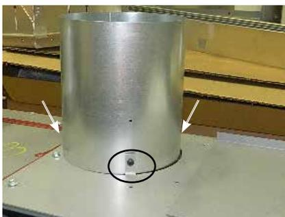
5. Connect the flex pipe to the adaptor with 3 screws.
