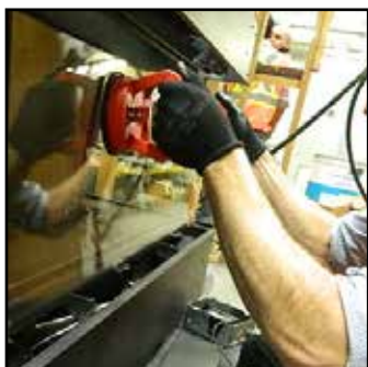
Handle glass with supplied vacuum clamps
