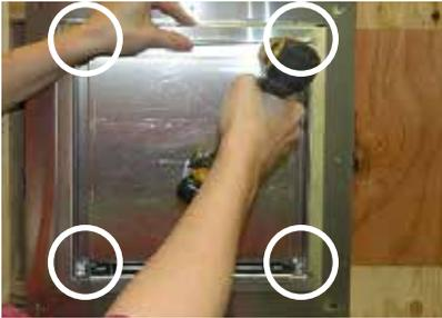
11. Loosen 4 screws in locations shown below, lift rain guard off screws (key hole slots).
