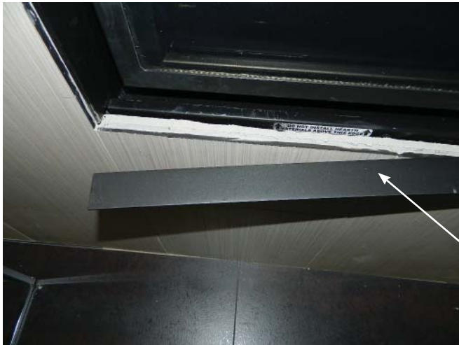
Figure 101: Top View - Sliding trim into place
