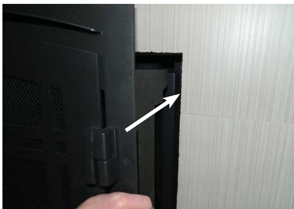
Figure 98: Line up Tabs with slot on Unit
