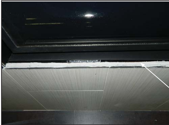
Figure 100: Top View - exposed non combustible materials
