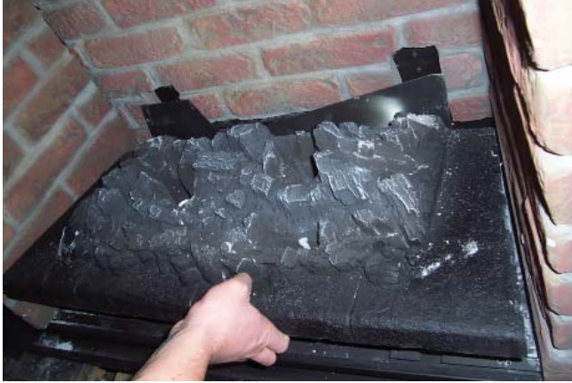
Figure 79: Burner Removal
