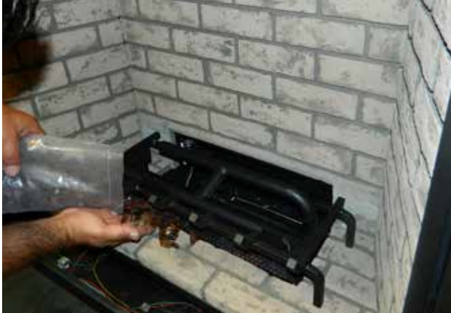
Diagram 3—Install Glass
