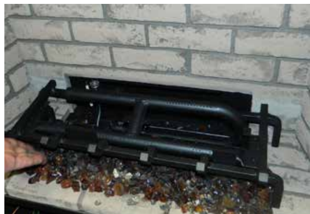
Diagram 4—Install Vermiculite + Lava
