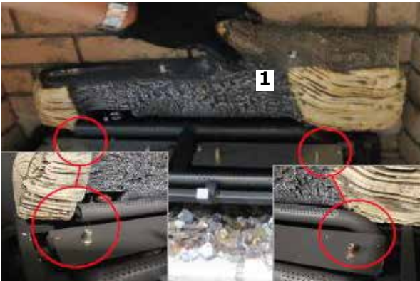
Diagram 7—Log 1 installation
