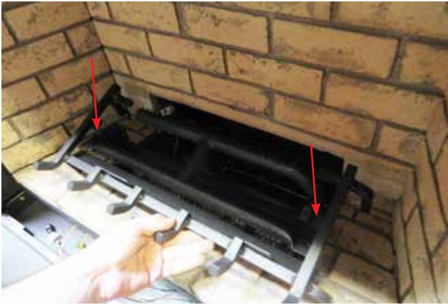
Diagram 2—Log Grate Install
