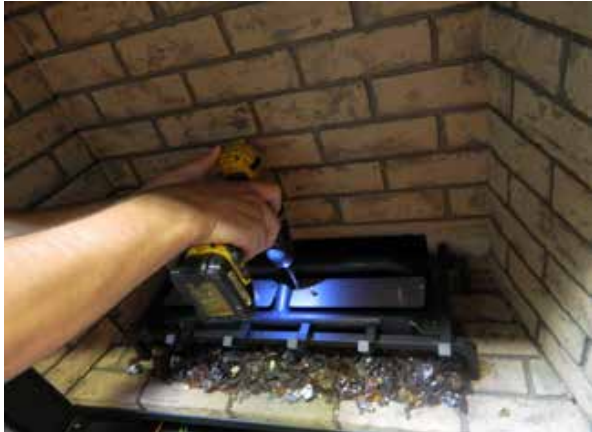
Diagram 5—Install Log support plates
