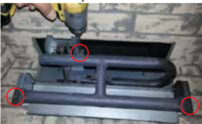
Diagram 2: Slide burner assembly to the right—then remove.
