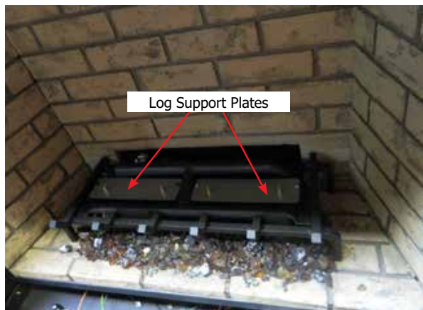
Diagram 6—Log support plates installed
