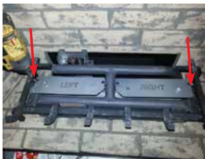
Diagram 1: Remove the left and right screws.
