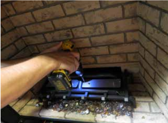
Diagram 5—Install Log support plates
