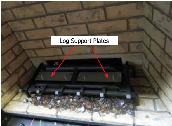
Diagram 6—Log support plates installed
