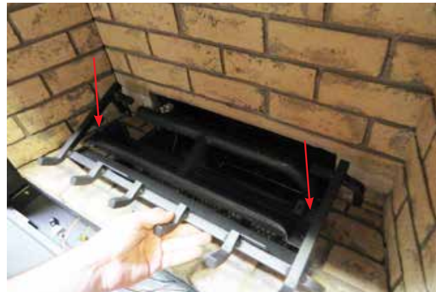
Diagram 2—Log Grate Install
