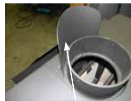
Installed Pipe Shield
