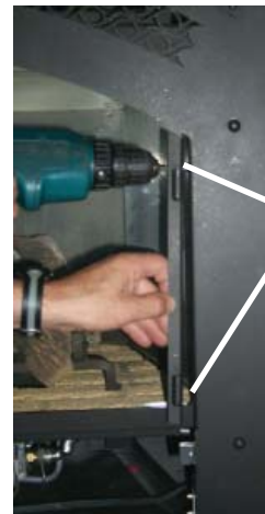
Door Bracket attaches with 2 screws.
