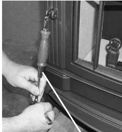
Secure using 7/16" socket wrench.
