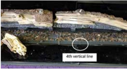
14. Install Log 8 - the left end of the log should sit 1" from the edge of the panel. The right end of Log 8 should be 2-1/2" from the right edge of the burner.
