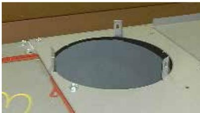
4. Connect pipe adaptor with 3 screws (use the lower holes on the adaptor).
