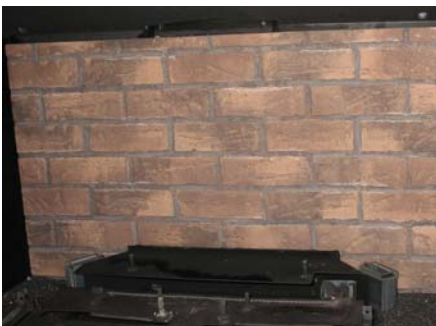
Back Panel Installed
