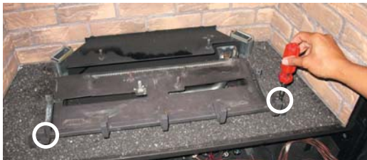
Diagram 1: Remove the left and right screws.
