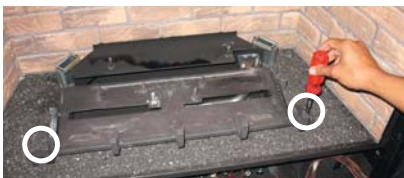
Diagram 1: Remove the left and right screws.
