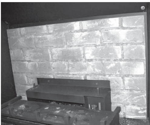
Back Panel Installed
