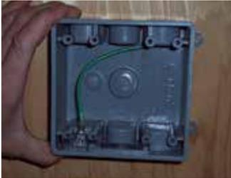
3. Remove center knock out from electrical box and install strain relief (strain relief nut not required).
