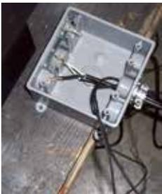
6. Attach low voltage wires to the switch - ensure to attach on the right side of the switch. This will make it easier to remove the 2nd battery terminal when replacing batteries. Fasten switch to right side of electrical box as shown below.
