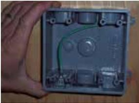
3. Remove center knock out from electrical box and install strain relief (strain relief nut not required).
