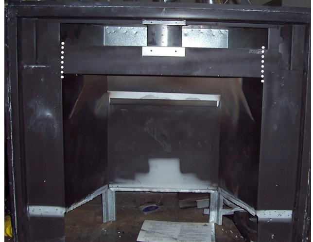
Cut out front cross piece to remove
