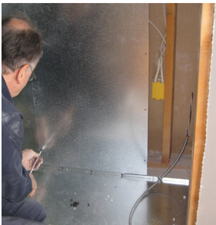
Fasten ZC box sections with provided screws.
