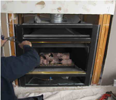
Remove unit from framing
