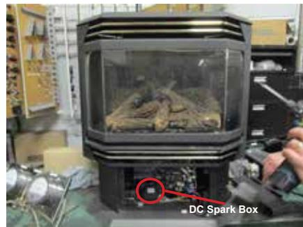
5. Open the battery compartment door on the DC spark box
