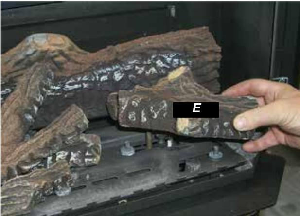
7. Place the notch in Center Log F over Log E and across the cut-out on Log A.
