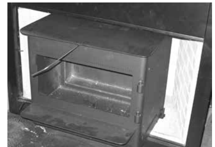
Diagram 5 Pull Rod In Place
