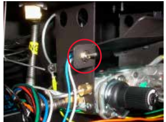
The Surefire switch is located above the valve. This can be accessed by removing the bottom louver/panel.
