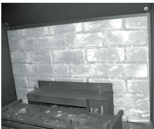
Back Panel Installed
