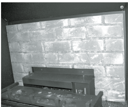
Back Panel Installed
