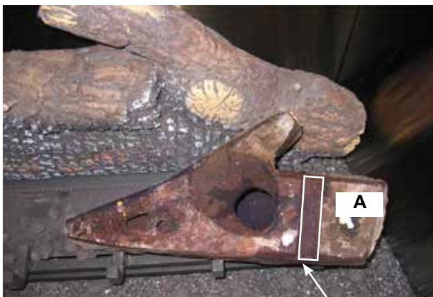
Notch location on underside of Log A (runs from back - front)
