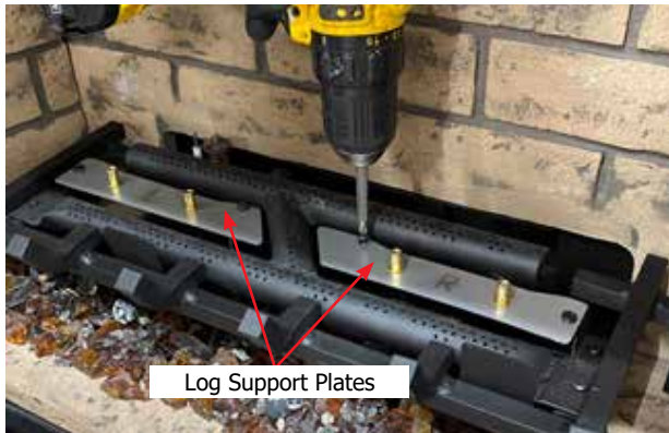
Diagram 5-Install Log support plate installation
