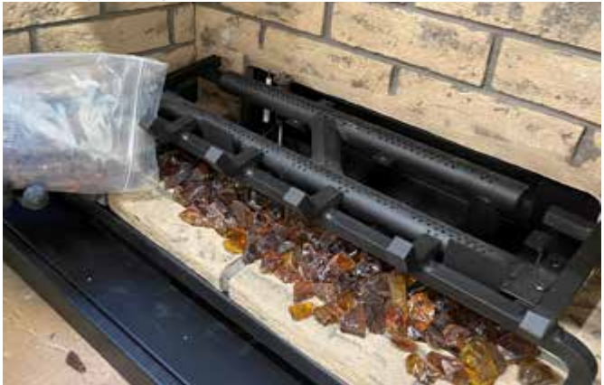
Diagram 3-Install Glass
