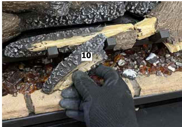
Diagram 15-Install Log 10
