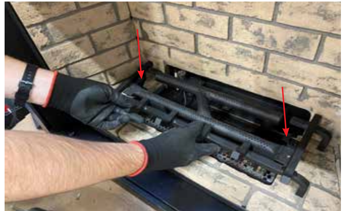
Diagram 2-Log Grate Install
