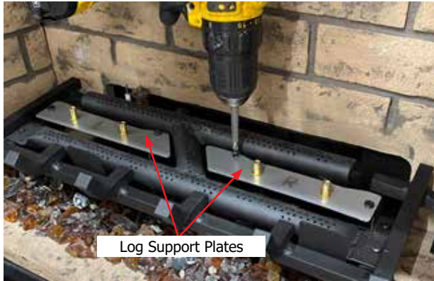
Diagram 5-Install Log support plate installation
