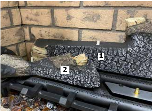
Diagram 7-Install Log 2
