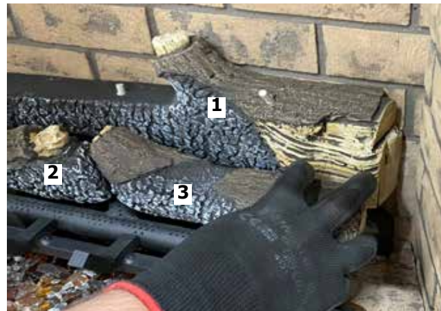
Diagram 8-Install Log 3
