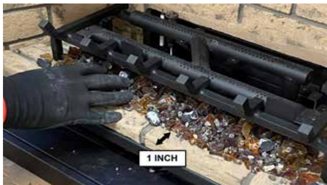
Diagram 4-Install Vermiculite + Lava
