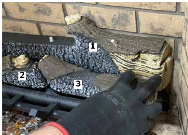
Diagram 8-Install Log 3
