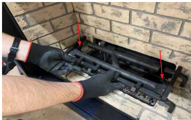
Diagram 2-Log Grate Install
