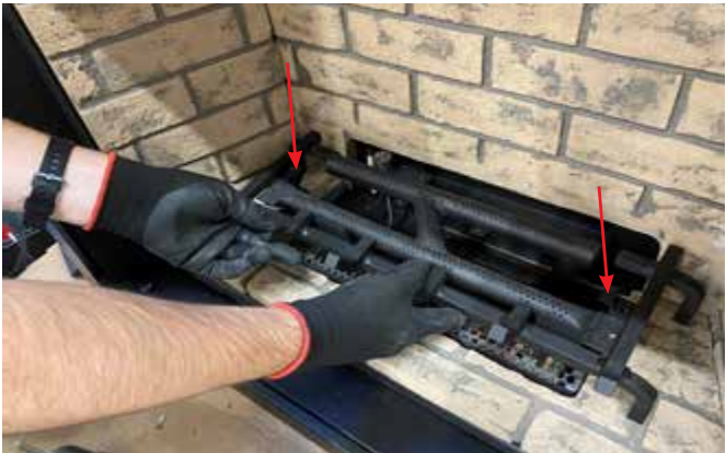
Diagram 2-Log Grate Install
