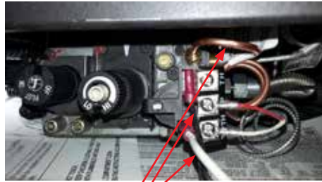
Diagram 4 Switch wires
