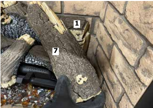
Diagram 12-Install Log 7
