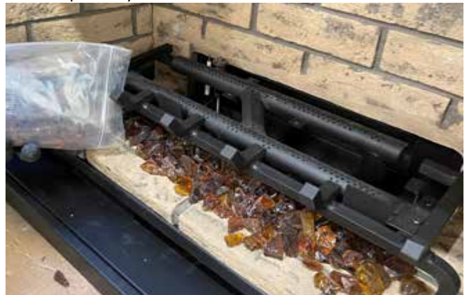
Diagram 3-Install Glass
