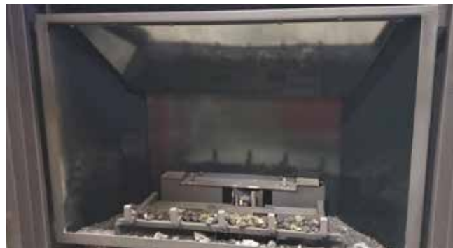
Diagram 7 - Completed Panel Installation
