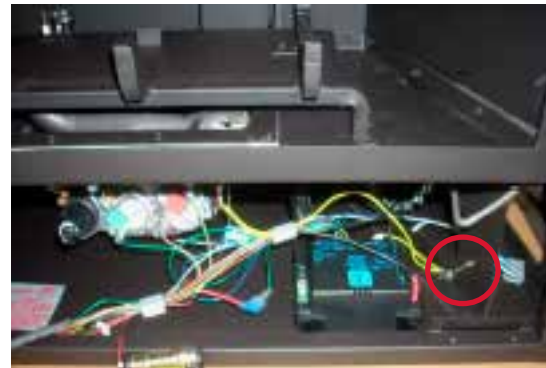
The Surefire switch is located in the left corner of the bottom louver/panel.
