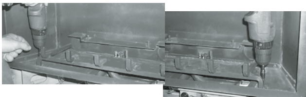
Diagram 1: Remove the 2 screws to remove burner.
