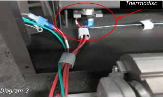
Fan control module is located on the right hand side of appliance if facing it from the front. Shown with metal cover removed. The fan control will be held in with 2 screws. The FCM COM wire would need to be disconnected also if the fan control module needs to be replaced.
