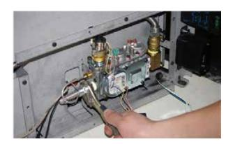
5) Disconnect the Pilot Supply Line from the Gas Valve
