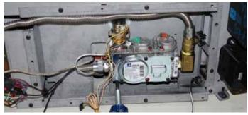
2) Loosen both screws at the top of the valve about ½ way out. Lift the valve body and lean outward. The Valve Brackets will rest open as shown on the right.
