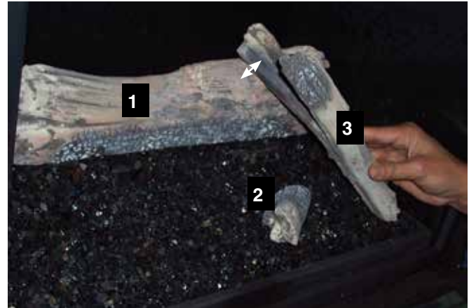
Line up pin locator and pin, Logs 1,3
