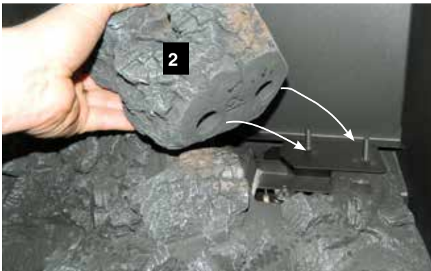
Log 2 pin locator, line up with pins on burner
