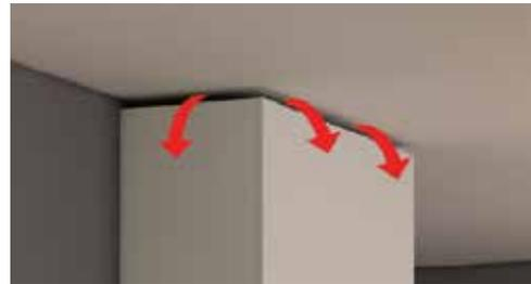
The ventilation opening may be fully open at the top of the enclosure. This type of ventilation opening would be used when the top of the enclosure is not visible from above and where the ceiling within the room is higher than normal. When creating this type of ventilation opening, measures should be in place to avoid having objects of any type falling or be thrown into the ventilation opening. Mesh screen or other preventative measures should be put in place.
