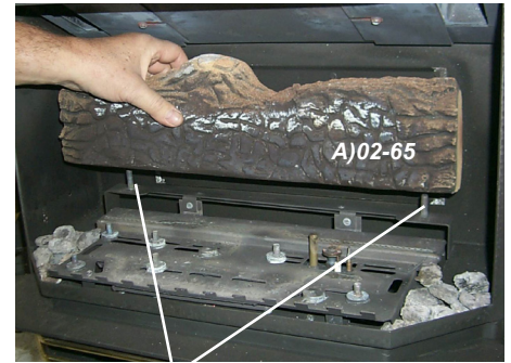
Pins on Rear Log Support
