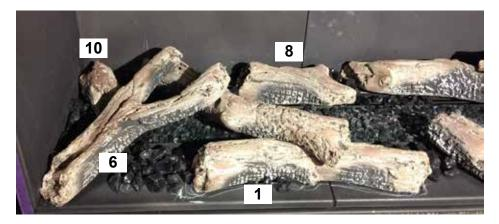
19. Install the 3.5 lb box of black charcoal glass (optional) or 1lb box of Andriron embers (optional) around the burner. **Make sure the burner surround is only 50% covered.**
