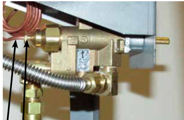
Diagram 3 Loosen nut to remove thermocouple
