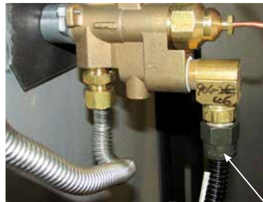
Connect flex line to valve
