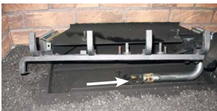
Diagram 2: Slide burner assembly to the right and then remove.
