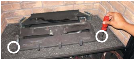
Diagram 1: Remove the left and right screws.
