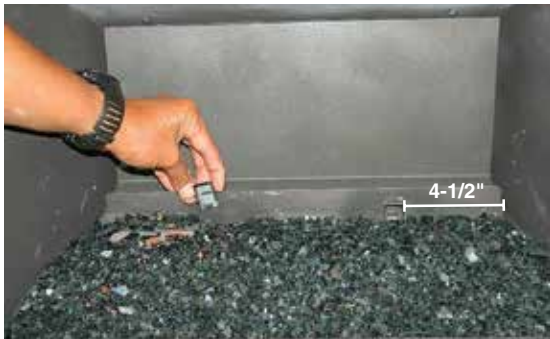
Log bracket install
