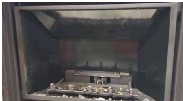
Diagram 7 - Completed Panel Installation
