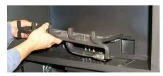
Diagram 1: Remove the left and right screws and then lift out the burner/grate assembly.
