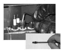
Remove burner orifice with a 1/2" wrench and discard. Use another wrench to hold on to the elbow behind the orifice.
