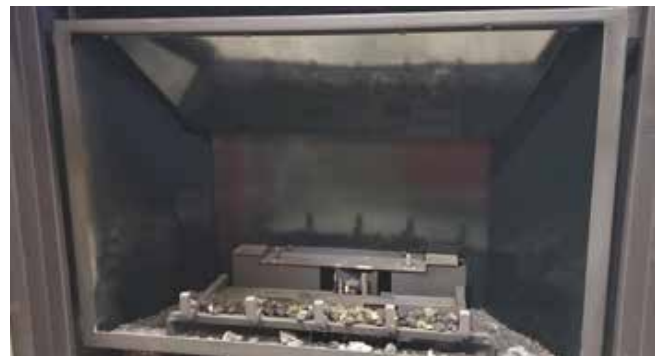
Diagram 7 - Completed Panel Installation
