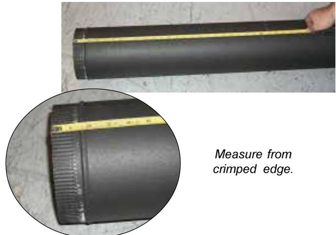
Measure from crimped edge.
