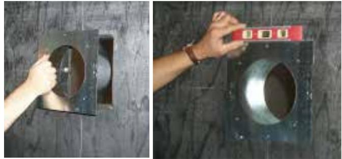
Wall Thimble - level & secure with 4 screws.
