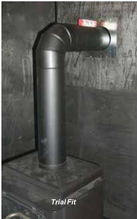
**NOTE: All joints, inner and outer must be sealed with Mill-Pac.**
