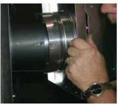
Note: The pipe seam should be facing down.
