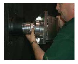
19) Apply Mill-pac to the exterior of the adjustable pipe section and fit the *Astrocap* over it and attach with 3 of the #8 x 13mm screws (stainless steel).
