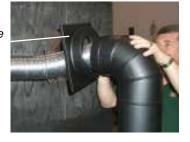
14) Slide both pieces of the adjustable pipe over the flex, the smaller dia. (male) section towards the elbow and the larger dia. (female) section towards the vent cap. Slide the flex and adjustable pipe sections through the wall thimble to the outside. The vertical pipe seams should be turned towards the wall.
