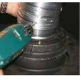
Fit flex over adaptor and secure with Mill-Pac and 3 screws.
