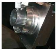
**18)** Attach the **Astrocap** to the 102mm dia. flex liner ensuring that the flex overlaps the collar of the vent terminal by a minimum of (35mm). Use Mill-Pac to seal and secure with 3 of the #8 x13mm screws (stainless steel).
