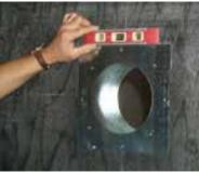
Wall Thimble - level & secure with 4 screws.
