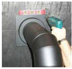
**25)** Install the trim collar over the starter collar and secure with a #8 x<sub>13</sub>mmscrew (black).
