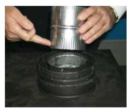
Adaptor into Starter Collar: longest crimped end into the Starter Collar.
