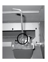
8. Put in the new LPG orifice with the Allen key. Then put back the pilot hood.
