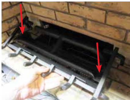
Diagram 1: Remove the left and right screws.
