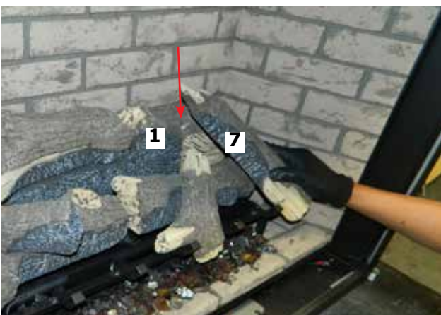
Diagram 13—Install Log 7
