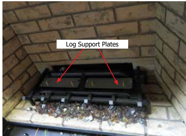
Diagram 6—Log support plates installed
