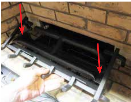
Diagram 1: Remove the left and right screws.
