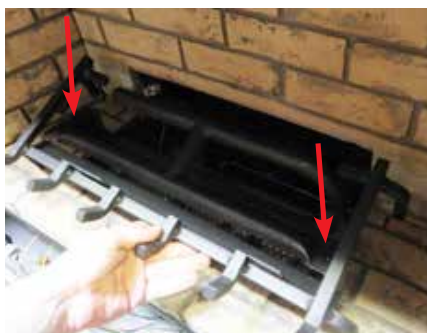
Diagram 1: Remove the left and right screws.
