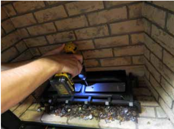
Diagram 5—Install Log support plates
