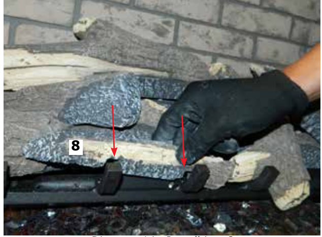
Diagram 14—Install Log 8
