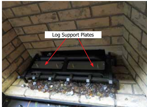
Diagram 6—Log support plates installed
