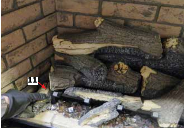
Diagram 17—Install Log 11
