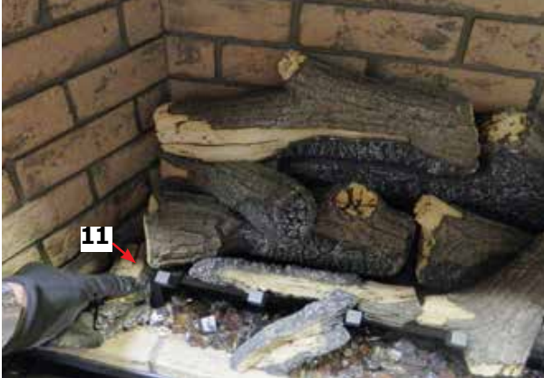
Diagram 17—Install Log 11
