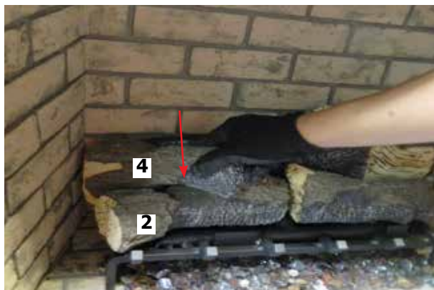
Diagram 10—Install Log 4
