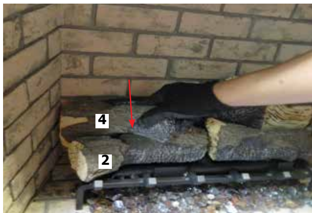
Diagram 10—Install Log 4
