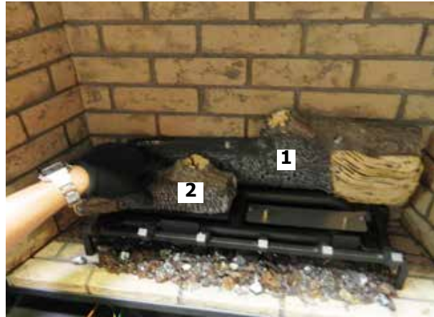
Diagram 8—Install Log 2
