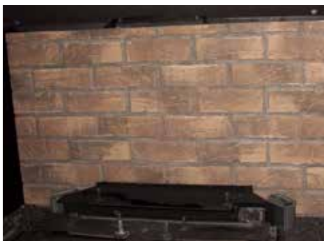
Back Panel Installed
