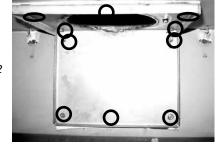
11. From the outside top of the firebox: install the intake collar assembly. Secure with 4 - 1/4" x 1/2" screws. Ensure all screws are tight, but do not over tighten. All 4 screws must be used.
