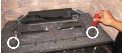
Diagram 1: Remove the left and right screws.
