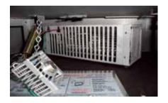
9) Slide the thermodisc/cover assembly onto the bracket clip on the left underside of the firebox. Ensure that no wires will touch hot surfaces.
