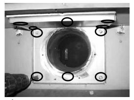
4. **From the outside rear of the firebox:** remove the intake collar assembly. Remove the 4 - 1/4" x 1/2" screws.
