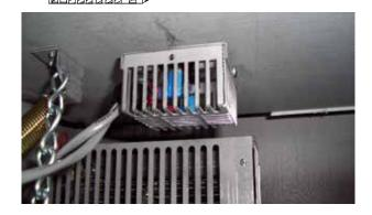
**10.** Install the Fan Control Module (FCM) on to the left side base of the unit and plug in to electrical receptacle in unit as shown.
