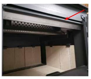
3. Incorrect Install: Return edge of smoke deflector seated under the glass wash.
