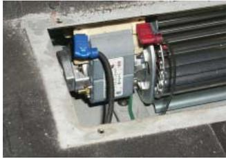
11) Remove the 2 screws from the fan bracket.
