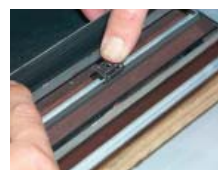
Push hold-down clip onto inside louver and press tab until it is at 90° to louver.
