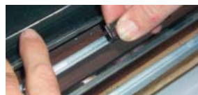
Push hold-down clip onto inside louver and press tab until it is at 90° to louver.
