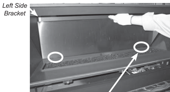
Right side back panel tab fitted into slot
