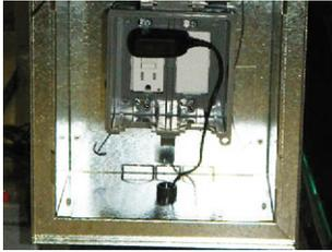
6. Run the AC adaptor wire from the recently installed electrical box, to the back of the unit end.
