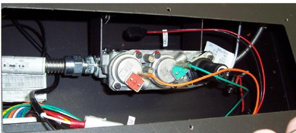
10. Remove 8 screws securing valve assembly.
