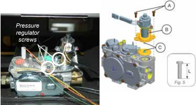
9. Re-attach the Pressure Regulator wire (disconnected in Step 6), and resituate the IFC, secure the screws that fasten the IFC Mounting Brackets.
