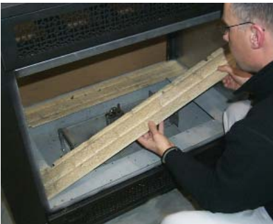
Remove the 2 Long Base Brick Panels
