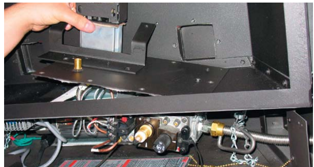
Diagram 5: Lift out Valve Tray Assembly
