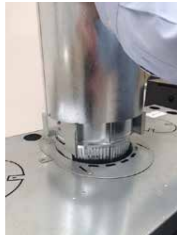
5. Air cooled bracket and pipe fitted to unit
