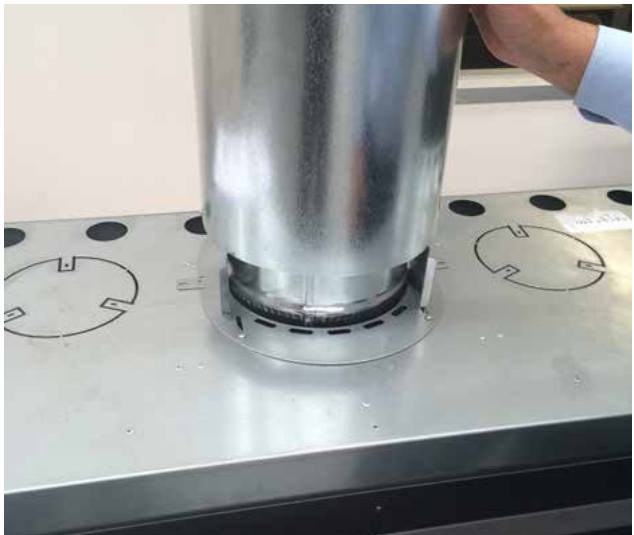
5. Air cooled bracket and pipe fitted to unit
