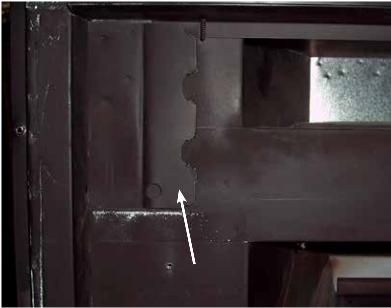
Flatten louver brackets
