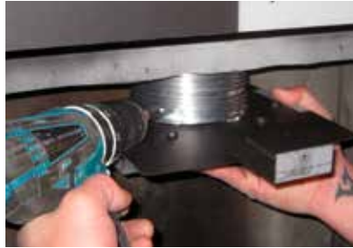
Secure vent slide plate to flex pipe with 4 screws/washers (supplied)
