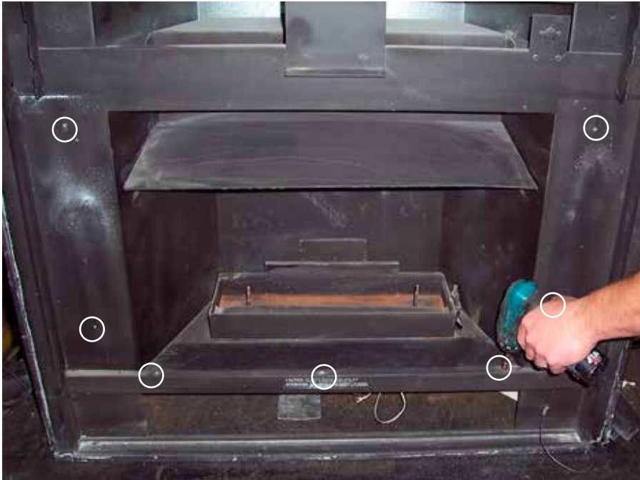
Remove 7 screws - remove Mesh Door Frame (if installed).
