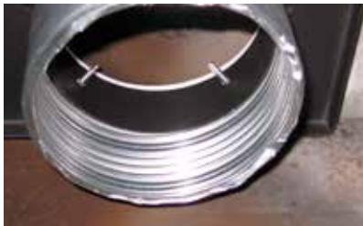
Diagram 1 Secure adaptor plate to existing Montigo firebox w/4 screws/washers (supplied)
