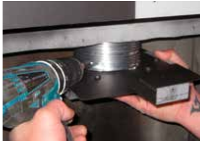
Diagram 2 Secure vent slide plate from E18E to flex pipe with 4 screws/washers (supplied)
