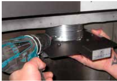
Diagram 2 Secure vent slide plate from E18E to flex pipe with 4 screws/washers (supplied)
