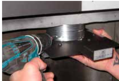
Secure vent slide plate from the E18E to the 4" (102 mm) flex pipe with 4 screws/washers (supplied)
