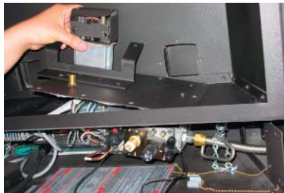
Diagram 5: Lift out Valve Tray Assembly
