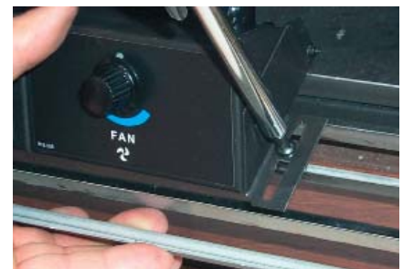
Secure right side with one screw.
