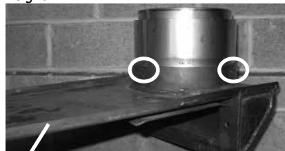
Diagram 2 Flue Adaptor
