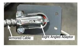
10. Install bracket onto side cover. Two holes may have to be drilled using a 1/8" bit prior to install, using the bracket as a template.
