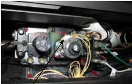
6. If fan installed—disconnect the "Com" wire from the valve.
