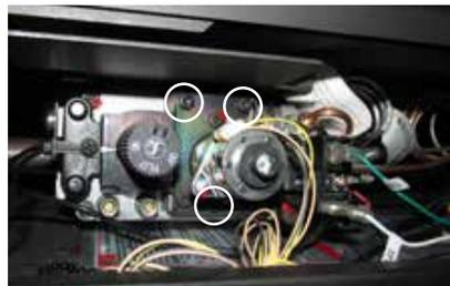
9. Pull off the pilot cap to expose the pilot orifice.
