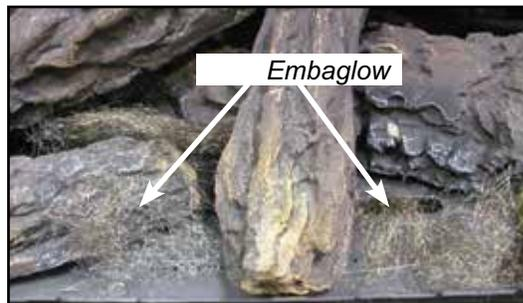
10. Next, take the white Platinum Ember material (provided) and gently separate the layers until you have a fine layer to place onto the Embaglow (steel wool type media).
