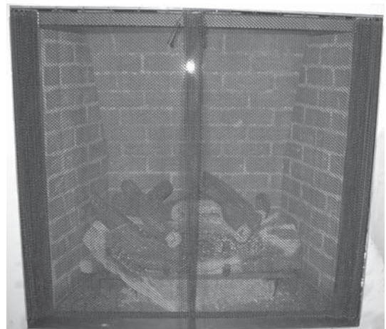
Completed Mesh Pull Screen Installation
