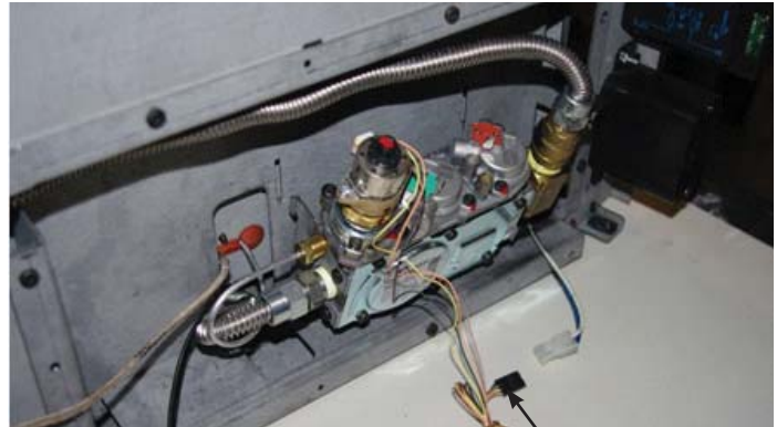
Cable from motor
