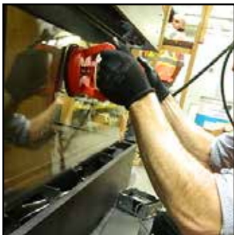
Handle glass with supplied vacuum clamps
