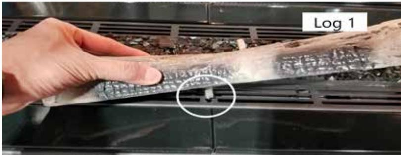
7. Lay the log on the firebox. Ensure the bottom left end of the log is 3/4" away from the edge of the firebox.
