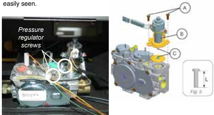
9. Re-attach the pressure regulator wire (disconnected in step 6), re-situate the IFC, and secure the screws that fasten the IFC mounting brackets.
