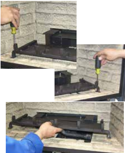
Diagram 1: Remove the left and right screws and then lift out the burner/grate assembly.
