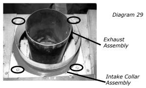
12. **From the outside rear of the firebox:** install the intake cover plate with 4 - 1/4" x 1/2" screws. Ensure all screws are tight, but do not over tighten. All 4 screws must be used.
