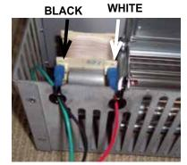
6. Position the fan base with the motor end towards the rear of the firebox and then slide the fan in towards the rear of the unit. Turn the fan housing slightly to the left and make the fan assembly parallel to the rear wall.
