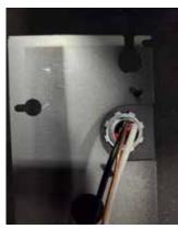
11. Connect the main harness wires (X1) to the armored cable using the 3 twist-on wire connectors provided. Make the connections according to color; neutral (white), live (black) and ground wires (green & bare copper) between the main harness (X1) and the armored cable.
