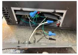
12. Tuck wires neatly into the unit using the cable ties and clip wire holder and re-install the side cover.
